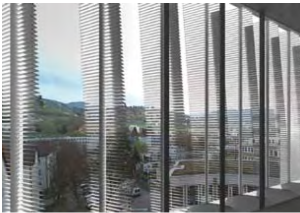
Fig. 1: Simulation model of the vertically rotatable sun-shading elements for the headquarters of Thyssen Krupp AG. The sun-shading elements can track the sun so that they both provide effective solar control and allow a good view of the surroundings.
