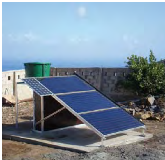
Fig. 2: Energy-autonomous compact system that was installed in November 2007 on Tenerife for seawater desalination. The daily capacity is about 120 litres.
