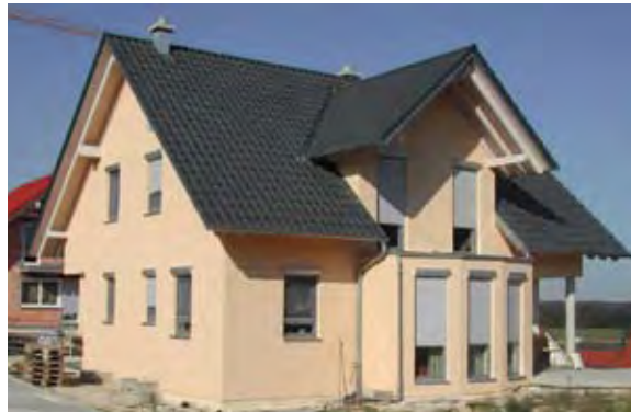
Fig. 2: Demonstration building (free-standing house near Giengen/Brenz) clad with the new VIP composite external insulation system (thickness 90 mm). Heat transfer coefficient (U value) of the wall, U_W = 0.13 \text{ Wm}^{-2}\text{K}^{-1} .
